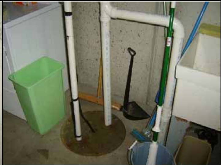
Replace cover and seal penetrations
