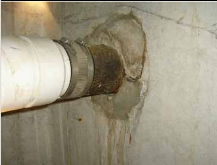
Replace mortar around pipe with hydraulic cement
