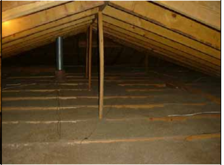
View of main gable in attic
