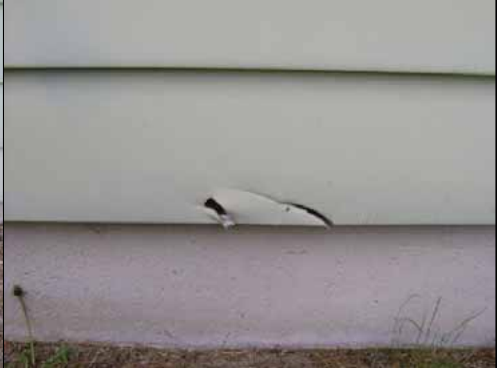
Siding damage
