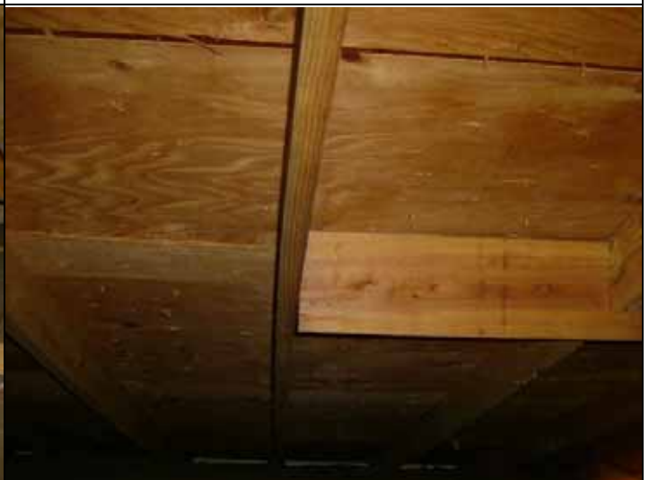
Termination of ridge on one rafter
