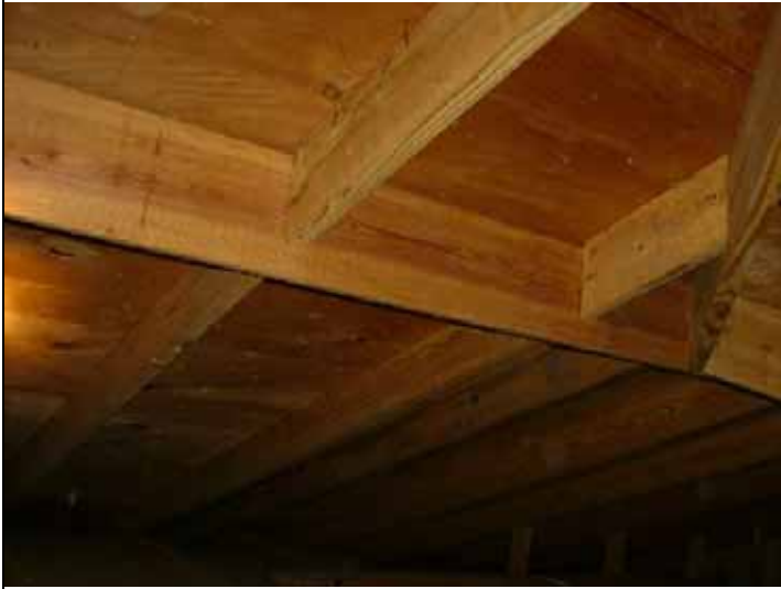
Another view of ridge and valley framing
