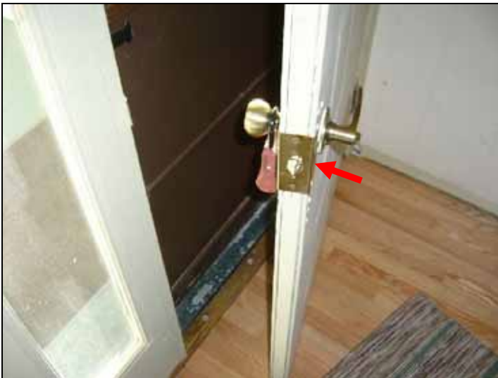
Repair to damaged door
