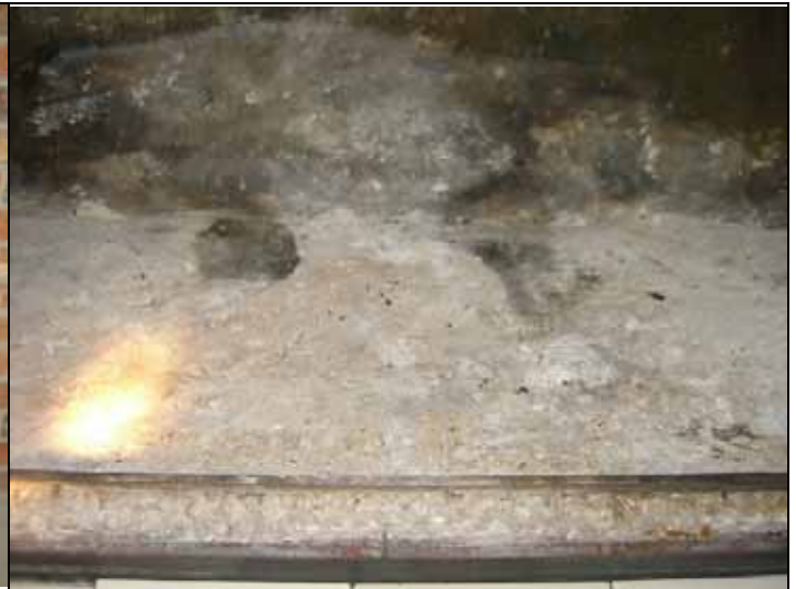
Firebrick deteriorated
