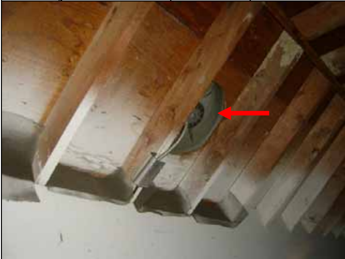
Attic vent fan in garage
