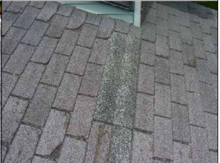
Deteriorated shingles
