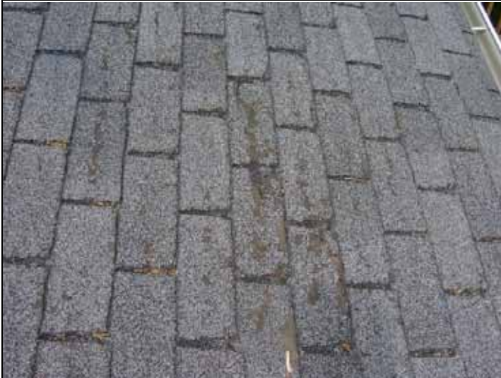
Deteriorated shingles
