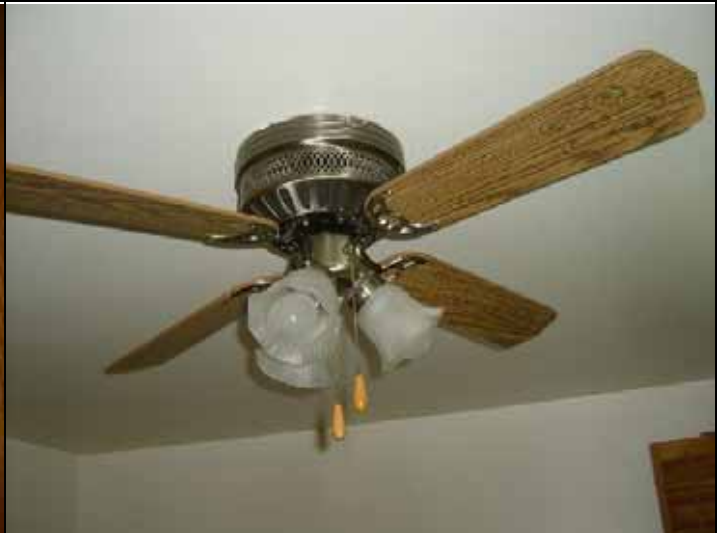
Typical fan, several rooms, wobbles and vibrates
