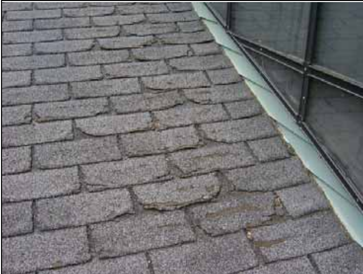
Deteriorated shingles
