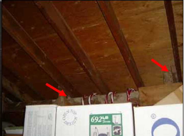
Splices above beam, roof rafters
