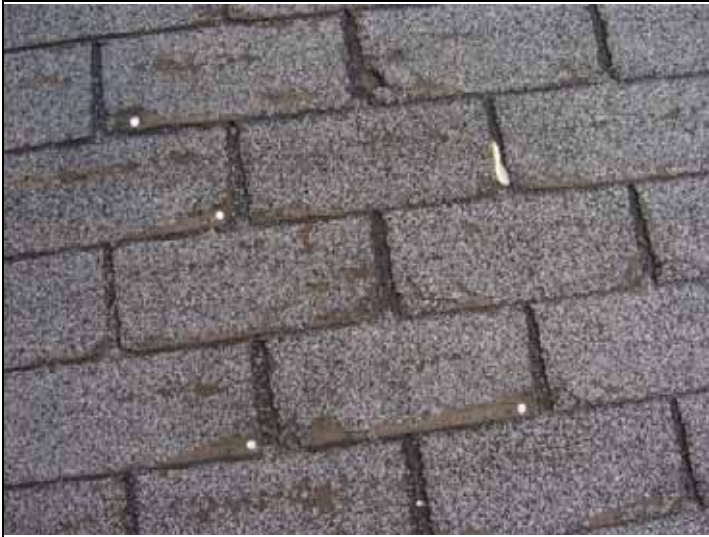
Deteriorated shingles
