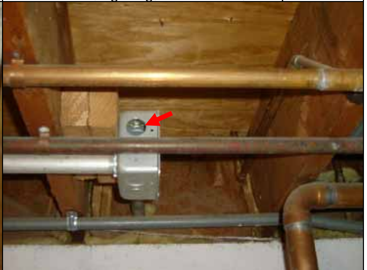
Knockouts missing
